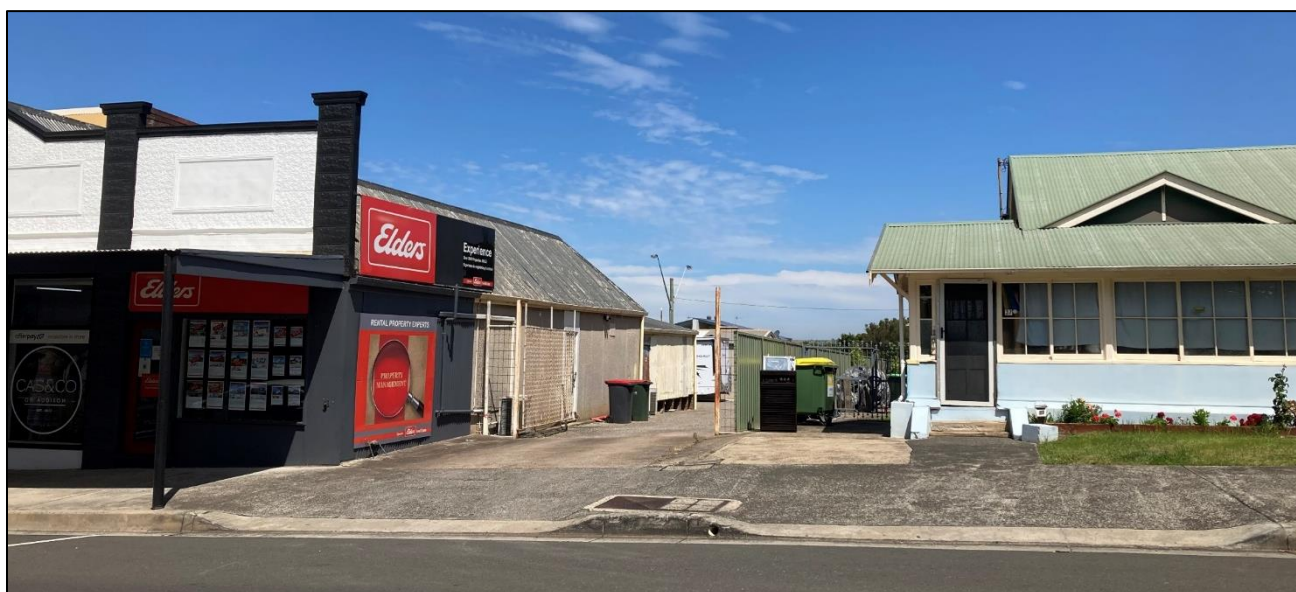
Figure 9: View of the heritage item and the dwelling to be demolished. Common boundary is shown by green dividing fence.
